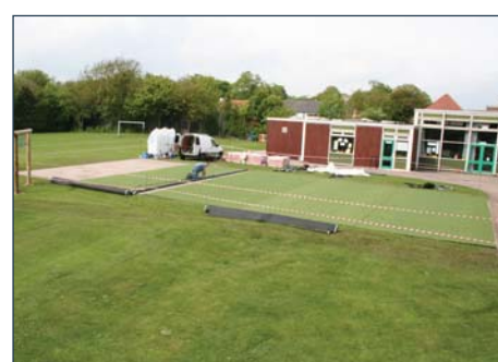
Installation of CitiGrass synthetic grass surface
