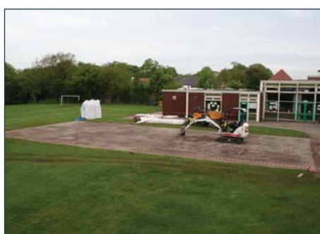
To improve drainage a stone raft is installed
