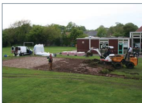
Work starts on the new CitiGrass Installation at Orston Primary School
